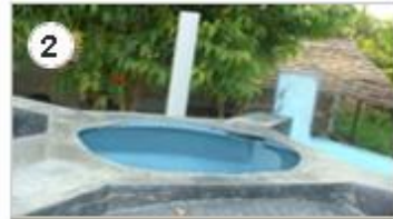
2 The first tank is the fermentation tank. Cattle manure is fed into it through an inlet.
