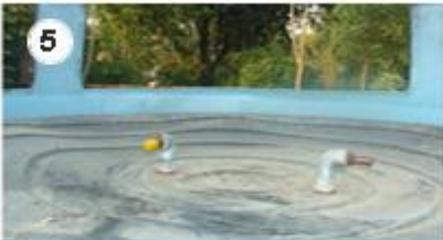
5 The gas holder tank connects to the household kitchen to provide biogas fuel for cooking. Meanwhile the residue of the manure is shifted to the slurry tank to be used as an organic fertilizer.
