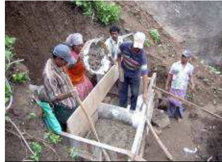
Sluice construction in Godiyapadu village/Photo credit: SOMNEED
