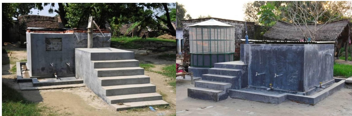
In Phase I of the project, 8 Gravel Sand Filters (left) and 3 Dug Well Filters (right) were built. Photo credits: BAMP
