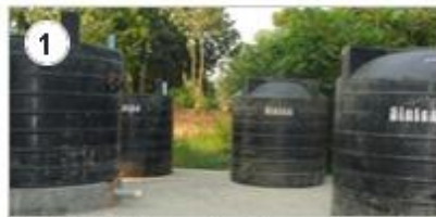
1 The Model Biogas Plant is a set up with four tanks, placed over ground. This enables temperature control in the system for steady production of biogas all year round.
