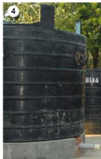
4 The manure in the fermentation tank gets stirred by a pump to avoid settlement, and for thorough decomposition. The decomposing manure then produces biogas, which is moved to the gas holder tank.
